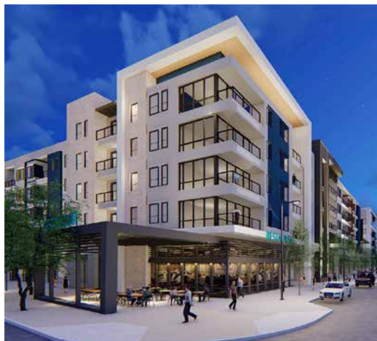
Top: Two new parking structures have been completed in Symphony Park, offering 1,300 spaces each, along Robin Leach Lane. (Image source: walterp Moore.com) Bottom: The Auric Symphony Park, a mixed-use development with housing and retail, is now open in Symphony Park. (Image credit: Southern Land Company)
