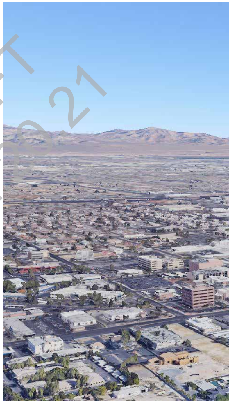
Google Earth image of the LVMD core, looking northeast. Charleston Blvd. runs east-west through the center of the image. (2020)
