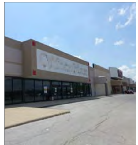
Above: A façade improvement program can help revitalize areas that have suffered from disinvestment. (Photo credit: Nicholas Eckhart)
