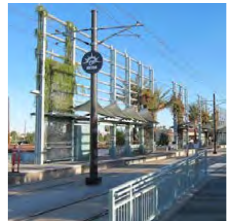
Top: Improved crosswalk, Denver, Colorado. Bottom: Valley Metro Rail station, Phoenix, Arizona.
