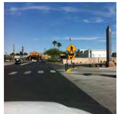
Top: Charleston Boulevard and Maryland Parkway. Bottom: University Road at the UNLV campus. (Photo credits: Nelson Nygaard)
