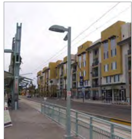
Top: Street utility upgrades taking place during streetcar line installation in Cincinnati, OH (Photo credit: Travis Estell)
