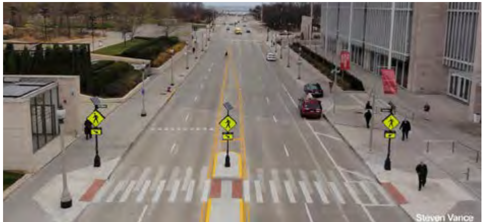
Top: Pedestrian activated crosswalk with accessible ramps and refuge median (Photo credit: Steven Vance)
